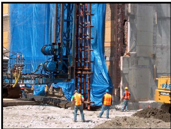
Figure 3 – Installation of Soil Mix Wall
