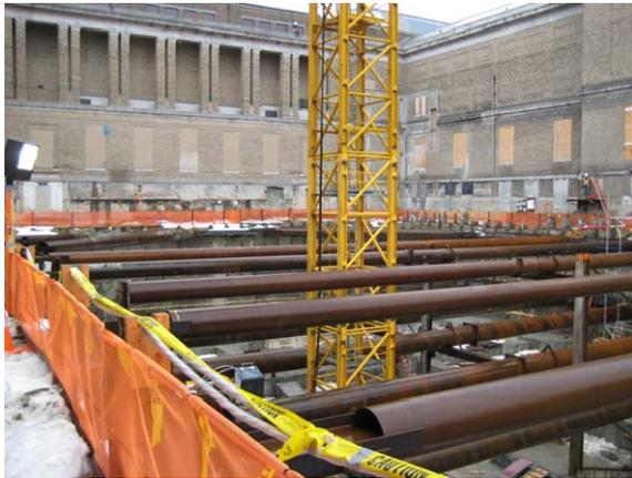
Figure 7 - Completed CDSM Wall and Bracing
