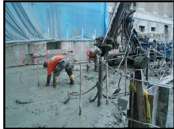
Figure 10 - Installation of Jet Grouting
