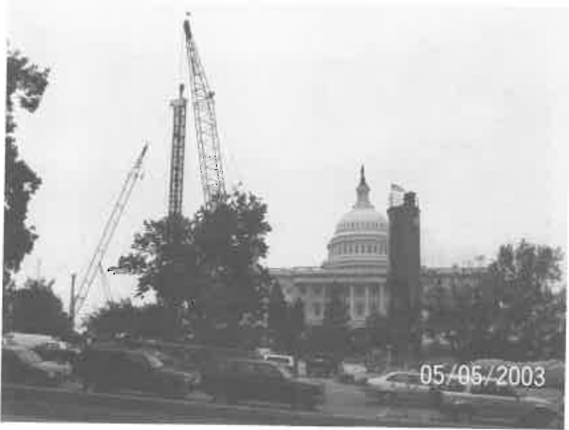
Figure 3- Deep Soil Mix (DSM) View with Capitol
