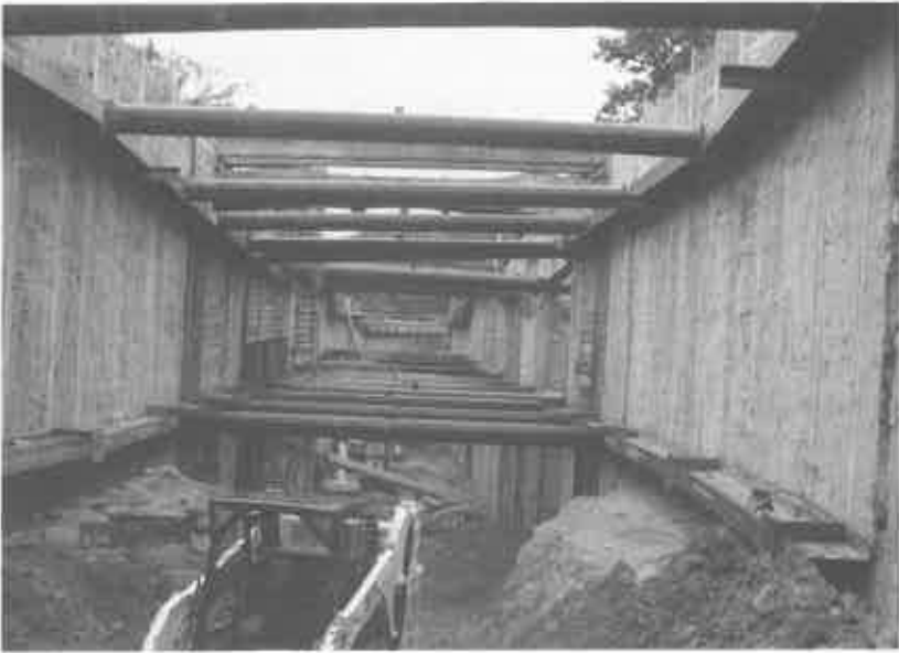
Figure 6 - Truck Tunnel Bracing at DSM
