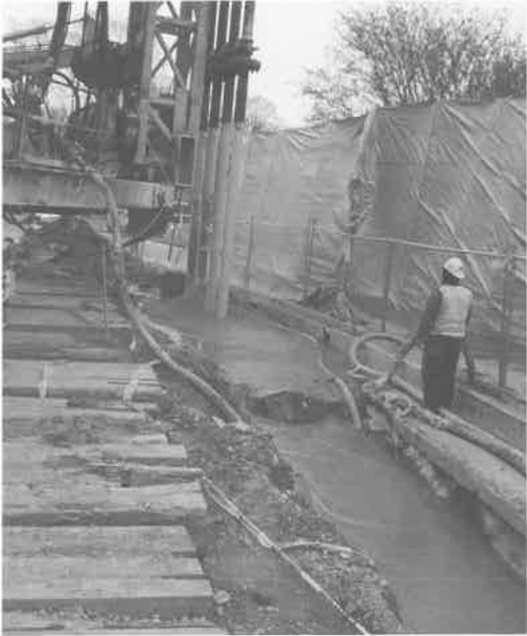
Figure 4 - Closer view of DSM Augers at Work
