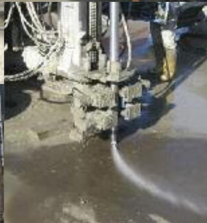
*This soil mix wall at Boston University required that the cutoff wall be extended beneath an existing duct bank. Jet grouting was used to complete the cutoff wall below the duct bank.*
