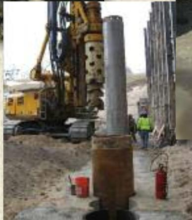
*Construction of secant pile wall showing concrete guide wall and drill rig with sectional casing.*
