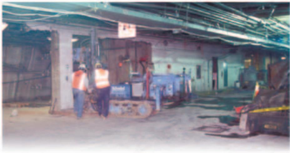
*During expansion of the baggage handling facility at Washington-Dulles International Airport in Virginia, micropiles were installed to transfer column loads to a deeper elevation and allow excavation below the terminal floor.*
