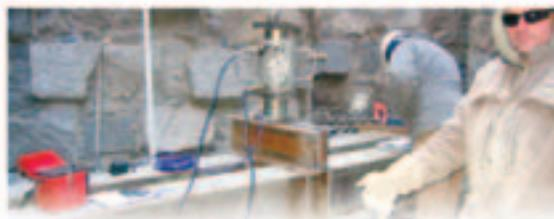
*Micropiles were used to increase the capacity of existing timber pile foundations during the expansion of the historic Trinity Church in Boston, Massachusetts.*
