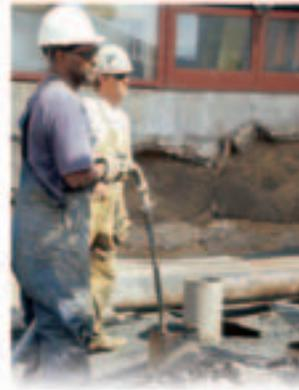
*Clockwise from top: Installing micropiles next to Children's Hospital in Philadelphia. Micropiles installed as soldier beams for excavation in difficult drilling conditions in Easley, South Carolina. Grouting micropiles. Micropiles used to support columns prior to excavation for a depressed railroad in Reno, Nevada.*
