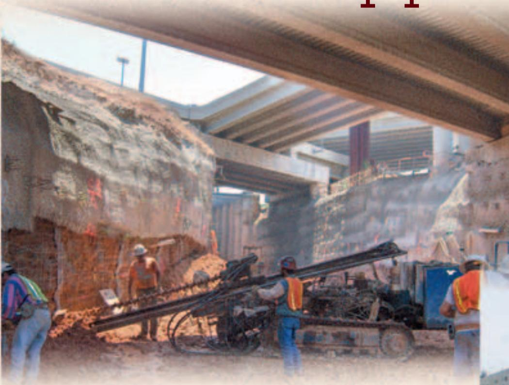
*Permanent soil nails were used to construct this excavation support system in limited overhead conditions.
