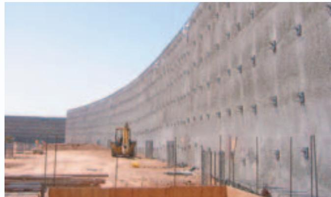
*This Panel Clockwise from Top: Part of the 192,000 square feet of soil nailing constructed to depress the railroad tracks through the center of Reno, NV; Permanent soil nail wall just prior to casting the wall face, Glendale, AZ; Design-build soil nail wall supports an excavation and adjacent structures, Berkeley, CA.*
