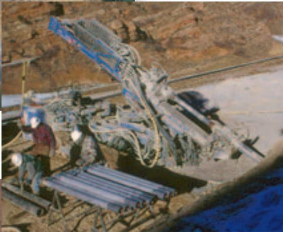
*Specialized down-the-hole hammers were required to install soldier beams in mixed rock and soil on this project in Tennessee (Top).*
