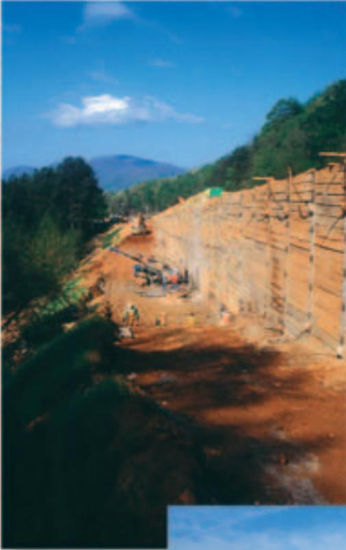
*A rotary drill installs tiebacks to stabilize a landslide below a highway – Georgia (Top).*
