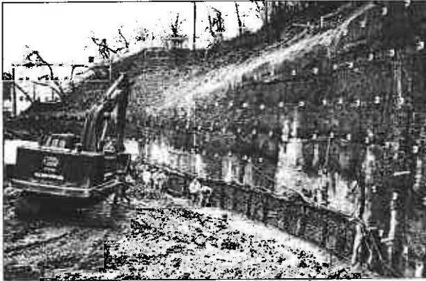
Figure 7 - Construction of Soil Nail Wall
