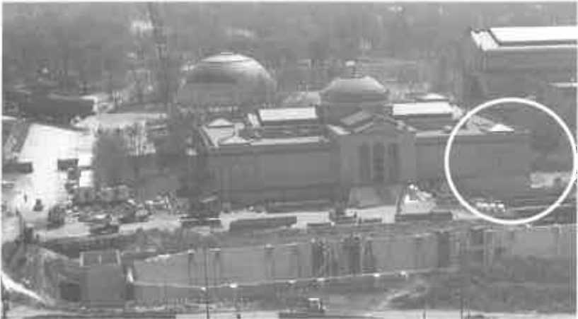
Figure 2: U-505 New Underground Exhibit and East Pavilion Underpinning Area (circled above)
