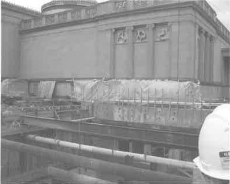
Figure 19: New Elevator & Stair CIP Walls Complete
