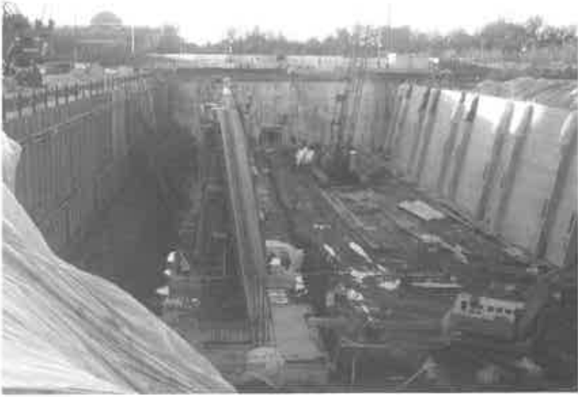
Figure 10: Sheet pile south wall - New Exhibit Area
