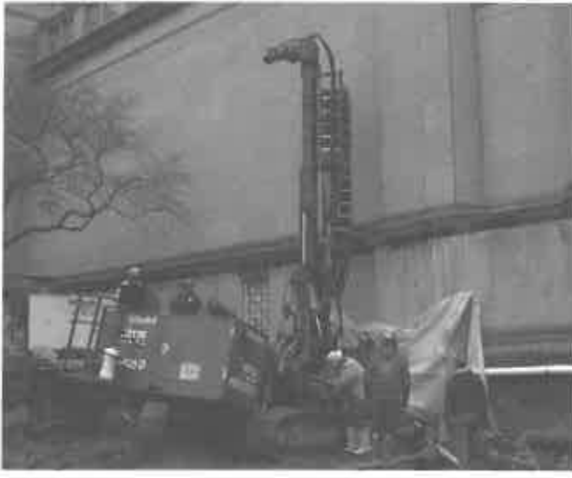
Figure 11: Installing Micropiles for PT Beam
