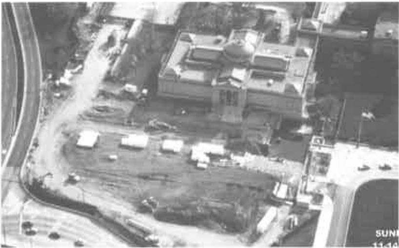
Figure 20: New Exhibit Area backfilled and Link roof water-proofing test underway
