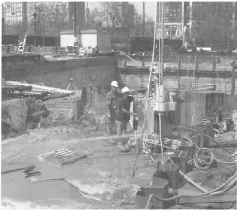
Figure 15: Jet grout test section - Link Area
