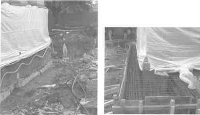
Figure 13: North Wall footing exposed (Left) and PT beam reinforcement (Right)
