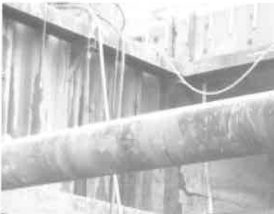
Figure 14: New Link and East Pavilion Area Excavation, Braces and Tieback Construction
