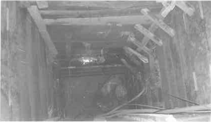
Figure 6: Underpinning Pier Construction
