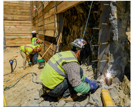
Welding of lagging studs
