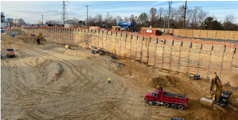
View of the retaining wall constructed using tiebacks
