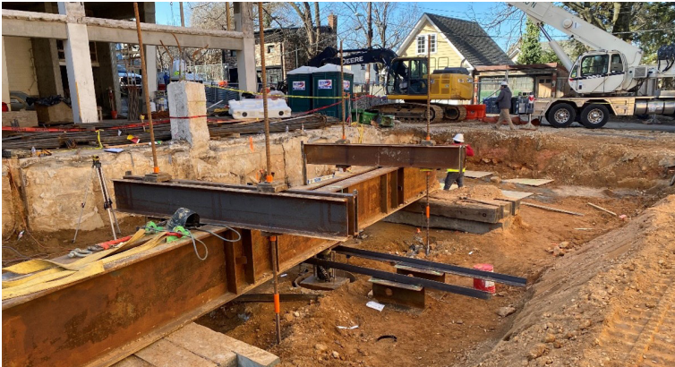
Modulus load test set up
