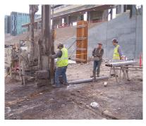
The drilling was performed using 7-5/8" diameter casing with j-teeth and a down-hole-hammer through 35 feet of undocumented fill consisting of sands, gravel, cobbles, boulders, and miscellaneous debris. Once bedrock was reached, the rock socket was advanced to create the bond zone for the micropiles.
