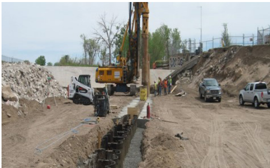
Sand Creek project, template construction
