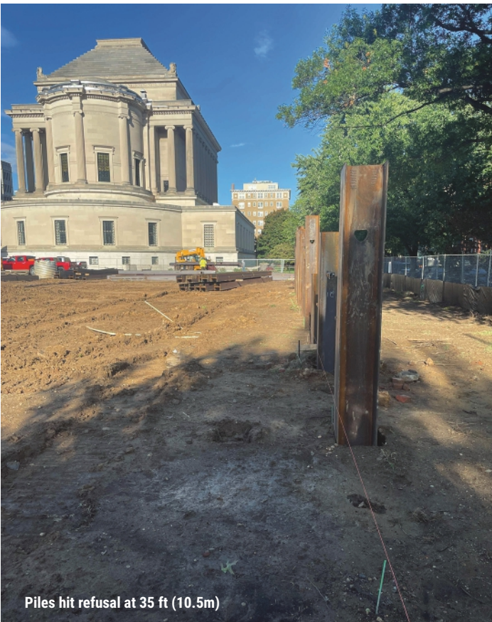
Piles driven to final depth
