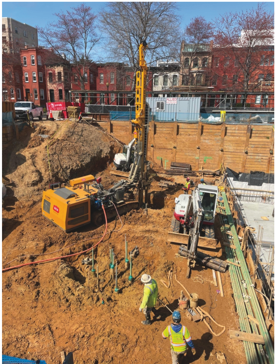
Micropile set up
