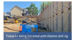
Lateral support was provided by 1 to 3 tiers of tiebacks. Tiebacks above the water table were installed with open-hole drilling and air flushing. Below the adjacent home and the water table, temporary casing and water flushing were used to maintain hole stability and limit ground and water loss. A Klemm anchor drill rig, cement silo, grout plant, and testing equipment were used to complete the tieback work.
