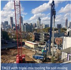
the required limits. The project proved that a soil mix cut-off wall could be successfully constructed in the Piedmont soils and limit deflections of nearby structures during dewatering without underpinning.
