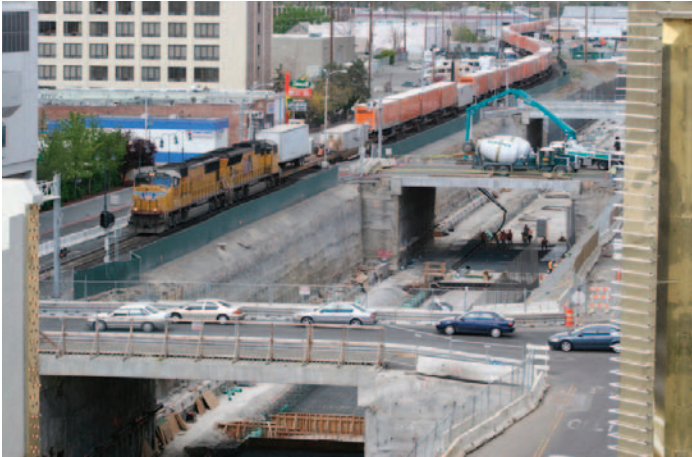
Figure 9. Soil nail shoring to protect railroad shoofly
