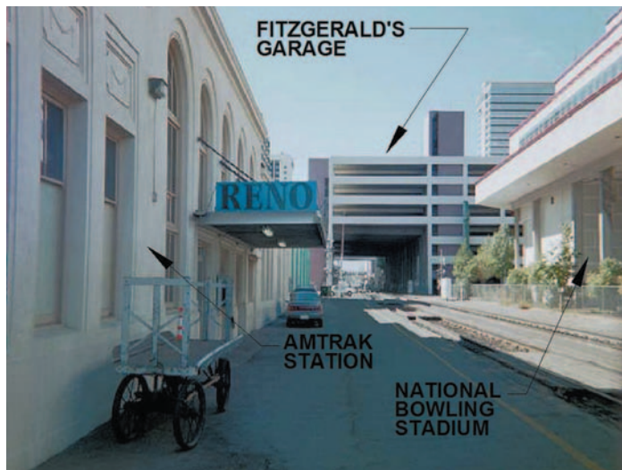
Figure 2. Preconstruction Condition Looking West
