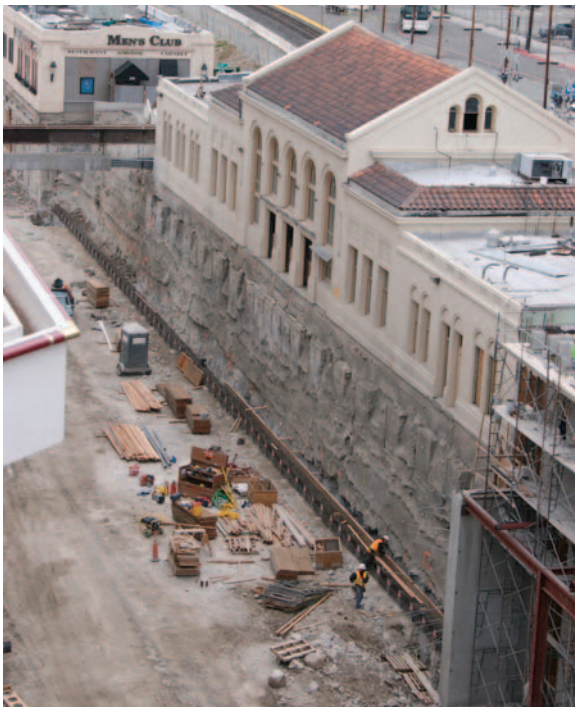
Figure 7. Micropile Underpinning of Historic Amtrak Structure
