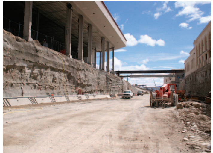
Figure 8. Micropile Underpinning of Bowling Stadium (left side)
