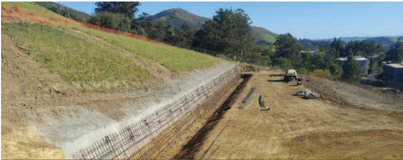
gallery wale construction
