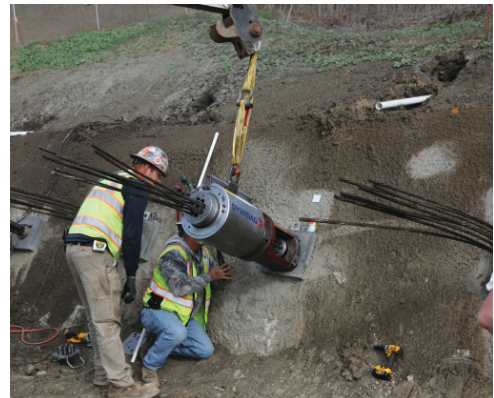
tieback testing
