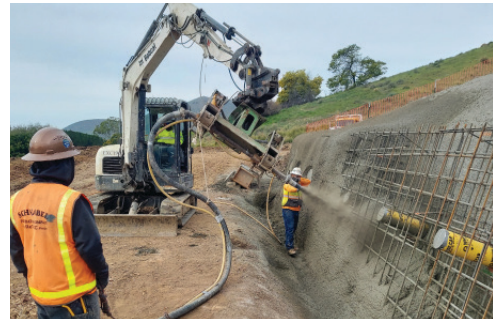
applying shotcrete to the gallery wale
