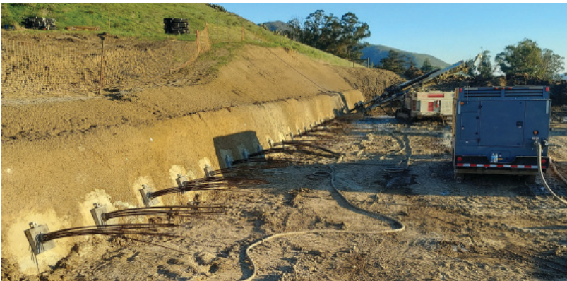
tieback drilling with 178 mm casing
