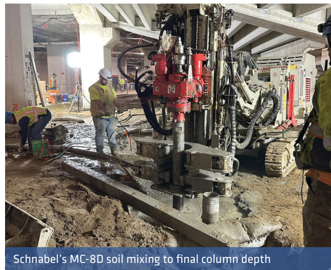
Schnabel's soil mix columns and waled hollow bar tiebacks
