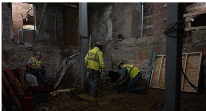
Schnabel's underpinning crew digging out a new underpinning pit in the Capitol Building's basement
