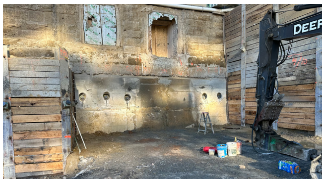
The connection between Schnabel's ERS and underpinning
