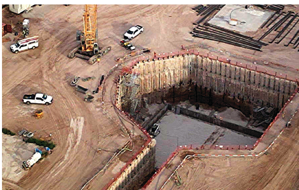
Completed IPS shoring cutoff wall, jet grout plug and tiedowns
