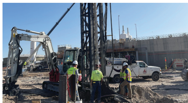
Installing tiedown anchors with CFA through the jet grout plug
