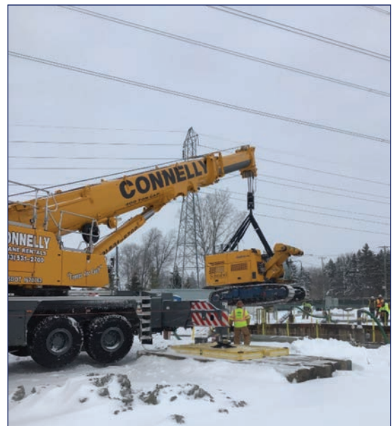
Fig. 3 Lowering base of rig into shaft
