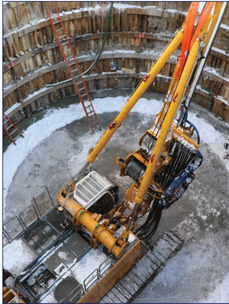
Fig. 4 Lowering lower mast into shaft
