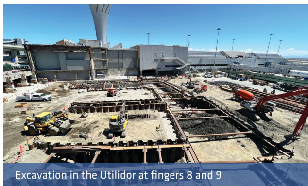
Installed foundation piles influenced the sheet pile clamping technique
