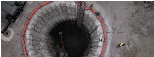
Aerial view of the launching secant pile shaft
