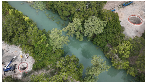
Aerial view of both secant pile shafts
