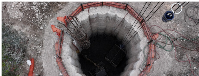
Aerial view of the receiving secant pile shaft
