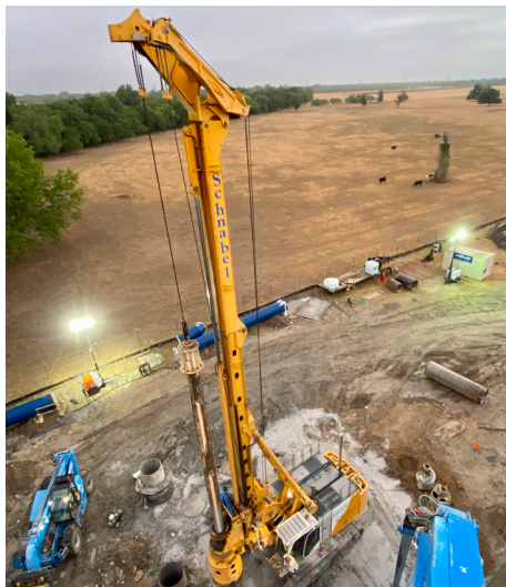
Schnabel's specialized Bauer drill rig equipment
