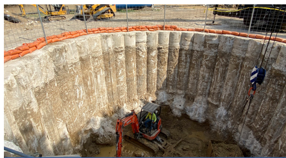
Schnabel team members excavating inside the launching shaft
