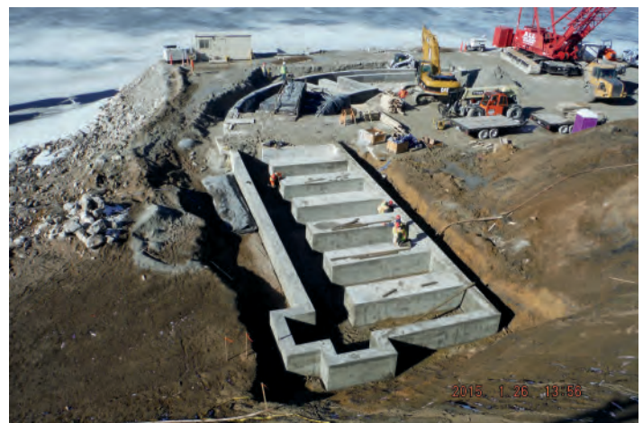
Guide wall for upstream diaphragm wall construction
