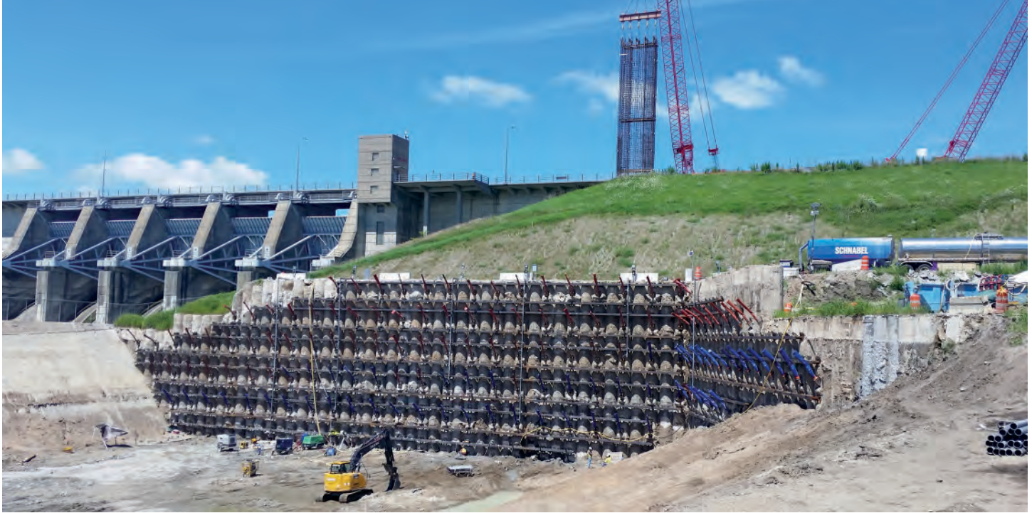
Secant pile wall for powerhouse construction (at front), with diaphragm wall cage being lifted for upstream placement (background)
